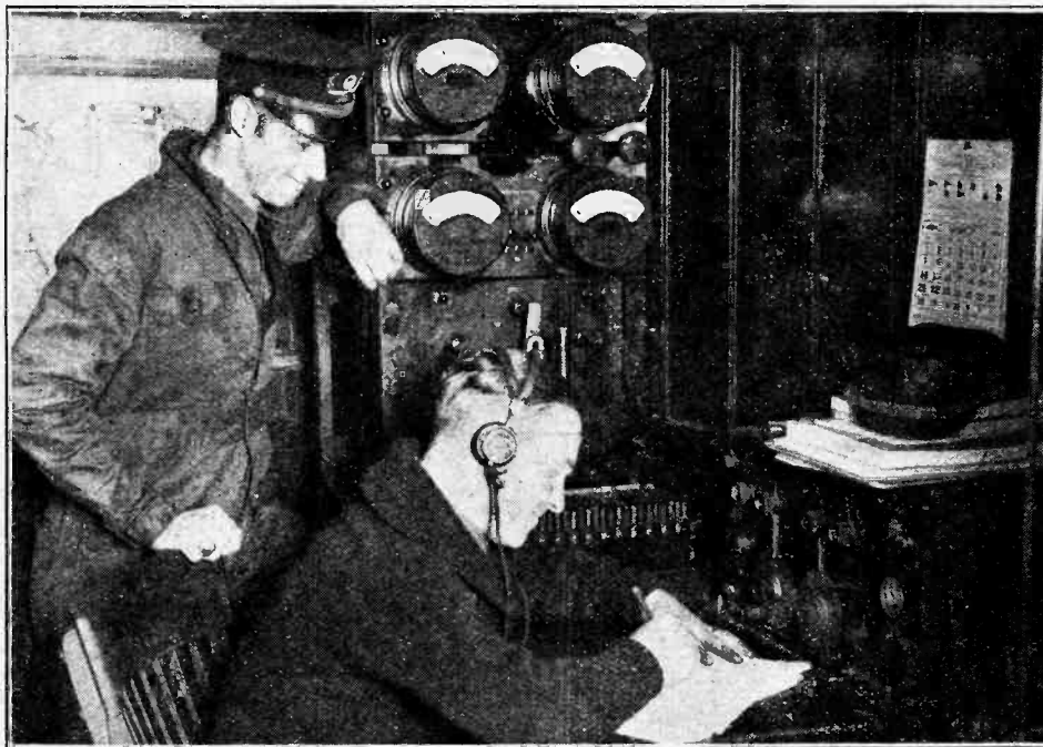
The commercial 1 kW. Marconi quenched-spark set of the "Chantier."
